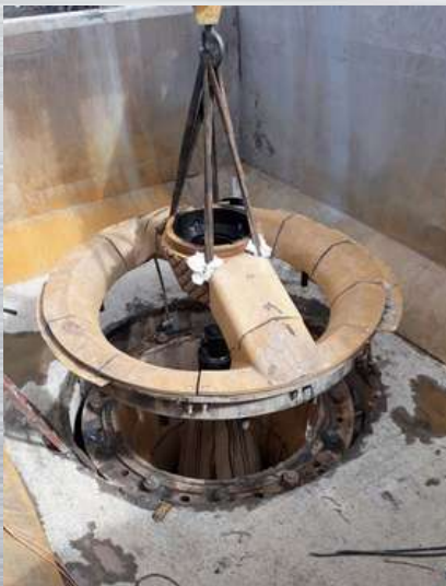
42-70 Gyratory Crusher Replacement
