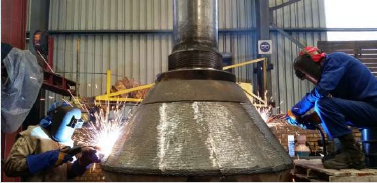
CH870 Head Centre Weld Repair
