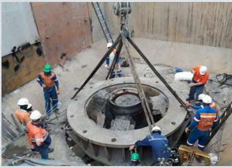
42-70 Gyratory bottom shell replacement
