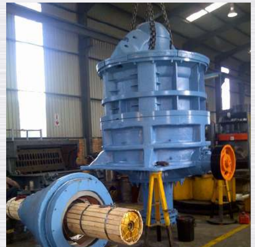
16-50 Gyratory Crusher Repair
