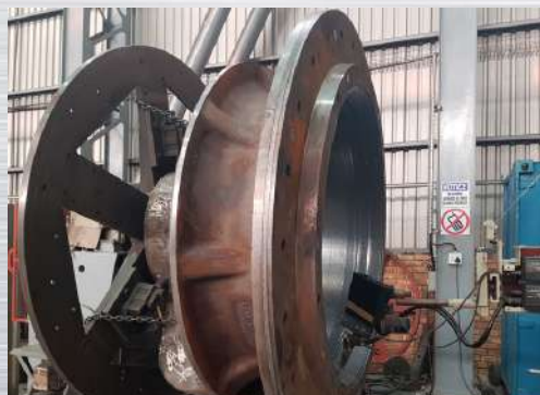
CH870 Top Shell SAW Repair
